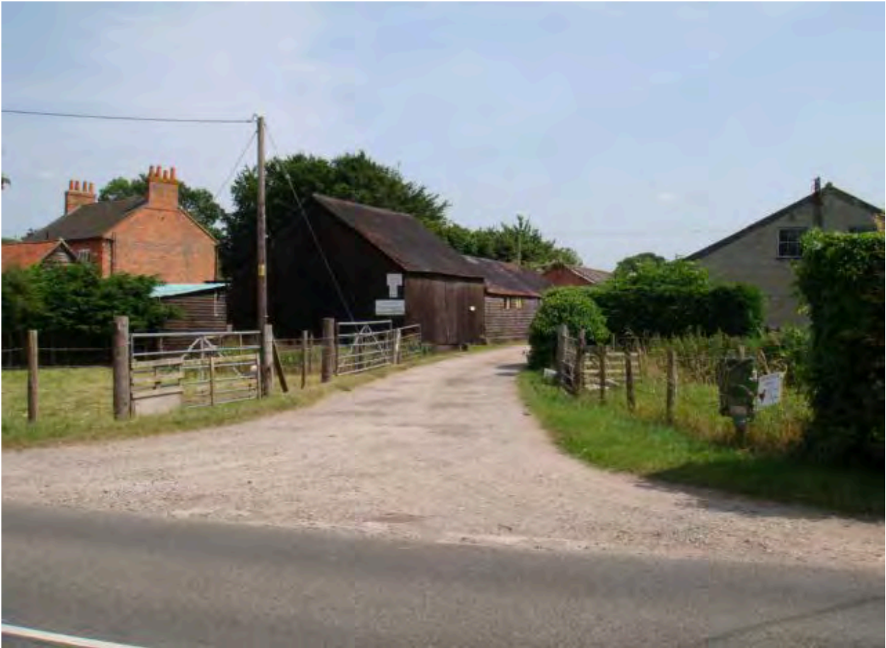
Photo 1: Frontage of riding school on Wallingford Road
